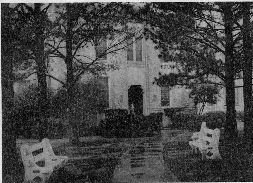
OLD STRUCTURE —The present Bry Hall on the Northeast Campus, has served as the Northeast library since 1939. Many students have passed under the pine arch through the doors of the "store-house of knowledge."
