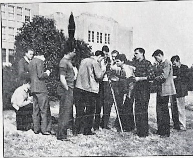
Under the supervision of John M. Chilton, instructor in surveying, the class is shown shooting the sun for latitude.
