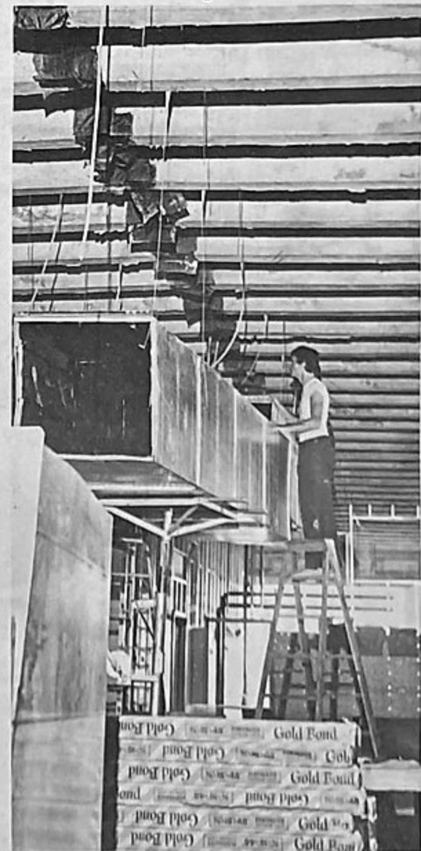
Walls in Stubbs Hall torn out
