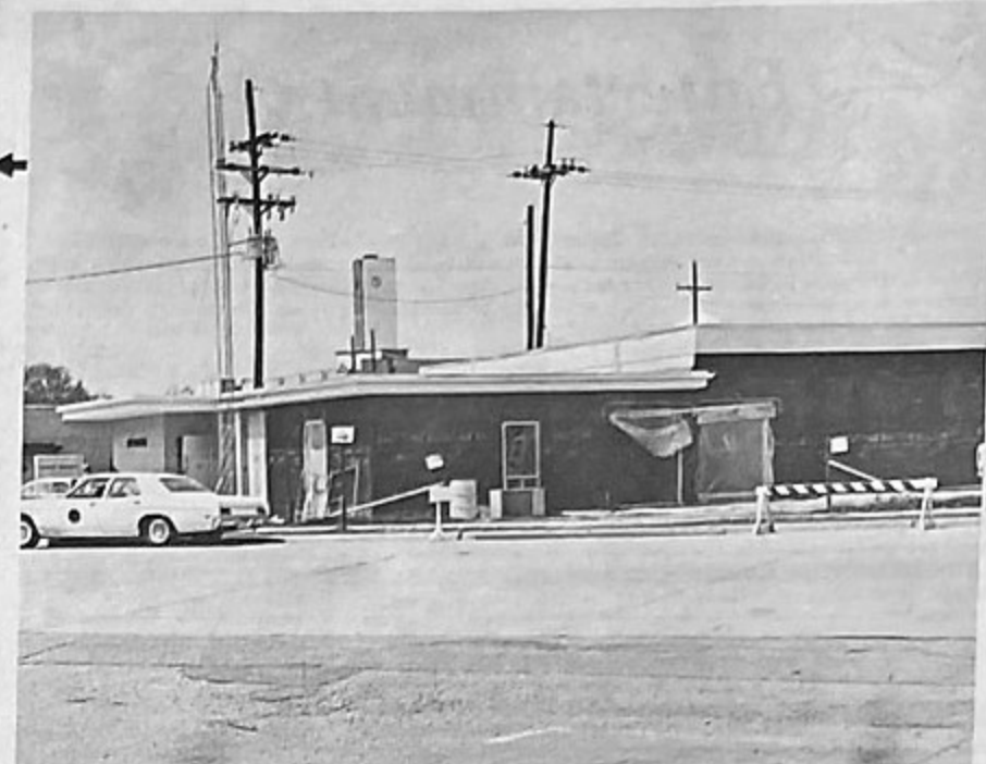
Post Office nearing completion
